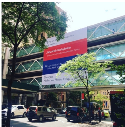
*New York Presbyterian Hospital の渡り廊下
